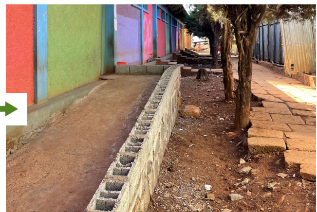
Fig. 11. Classroom entry (after). To improve accessibility, a ramp was installed to provide access to at least one classroom.
