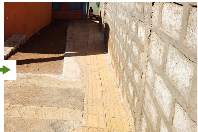
Fig. 9. Pathways (after). Accessibility of the pathways was improved by removing obstacles, creating clear pathways, and adding tactile paving surfaces.
