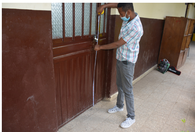
Fig. 60. No visual contrast. The dark brown doors blend in with the brown walls around them. The lack of contrast can be particularly challenging for people with visual impairments to differentiate between the door and the surrounding surface.
