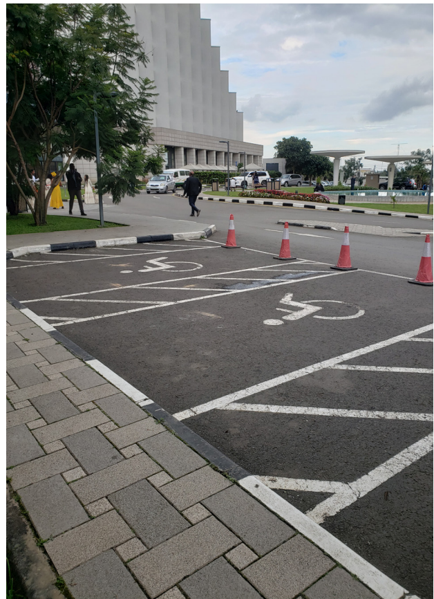
Fig. 39. Inaccessible parking. There is no curb ramp between the sidewalk and parking; the sidewalk is too narrow (<1200 mm) for wheeled mobility aid users; traffic cones block access to parking, and there is no vertical signpost.
