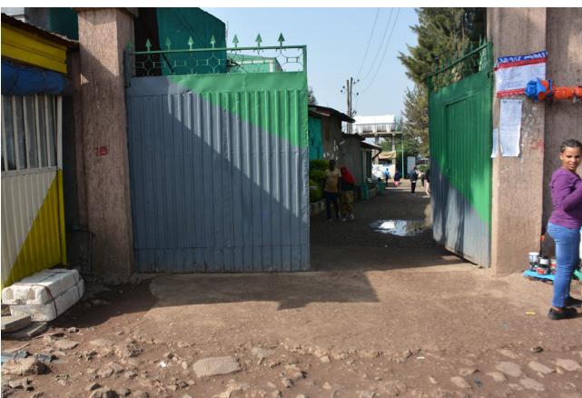
Fig. 57. Unsafe entrance. This entrance is used by both vehicles and pedestrians, creating safety risks for pedestrians. For improved accessibility, a separate entrance should be created only for pedestrians.
