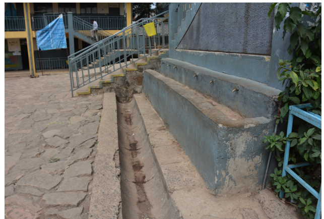
Fig. 81. Inaccessible wash area. No legroom, no color contrast and a large drainage system in front of the wash areas makes this wash area fully inaccessible.
