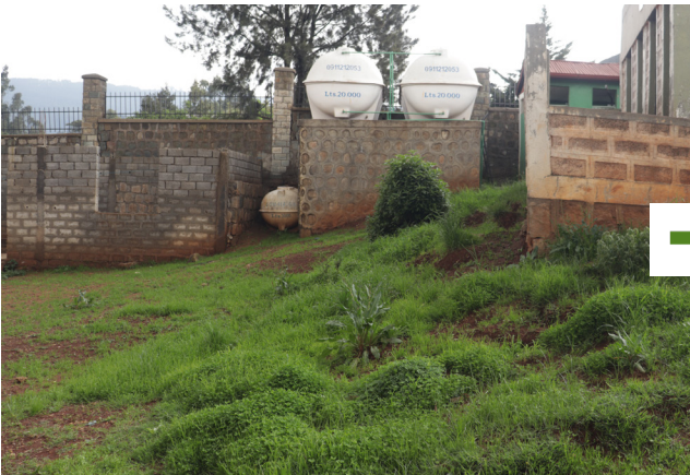
Fig. 6. Circulation (before). The entrance and circulation within the school's compound were inaccessible due to uneven terrain and lack of clear pathways.
