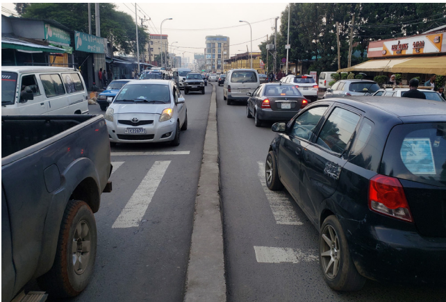
Fig. 33. Unsafe crossing. This crossing lacks a traffic island and curb ramps, posing a safety risk for pedestrians, particularly for people with mobility and visual impairments.
