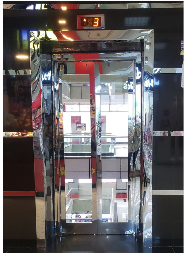
Fig. 73. Reflective elevator door. This elevator door has a highly reflective surface, which poses a significant challenge in distinguishing it from the door frame and the adjacent surroundings.
