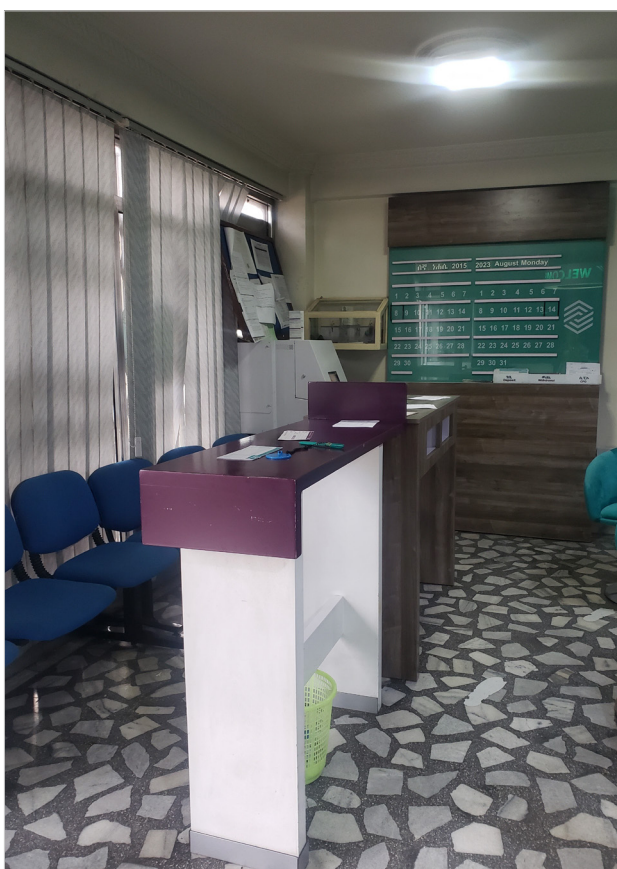
Fig. 68. Inaccessible waiting area. This waiting area is not accessible for wheeled mobility aid users due to insufficient maneuvering space. (less than 1500 x 1500 mm) Moreover, the table top is too high for wheelchair access (recommended height is 750–800 mm).
