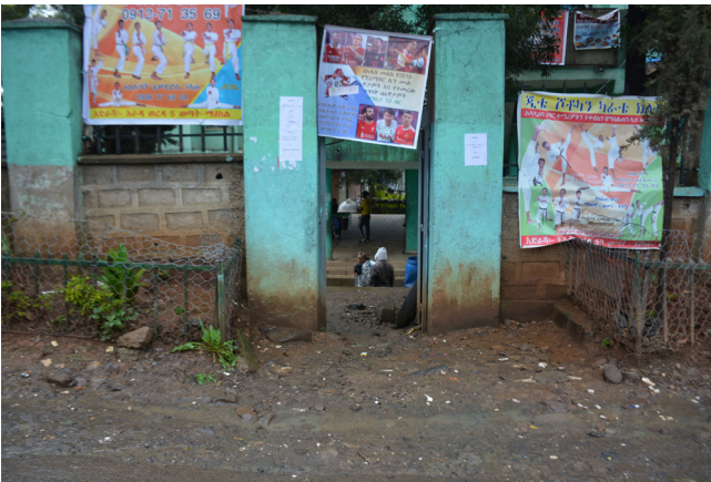
Fig. 56. Inaccessible entrance. This entrance is too narrow (<900 mm) to access with wheeled mobility aids; the path leading up to the entrance has an uneven surface; there is also a lack of visual and tactile cues.
