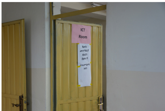
Fig. 61. Signage placement. Signs should not be placed on the door itself but on the wall of the opening side of the door to ensure that the sign remains clear and visible, even if the door is open.
