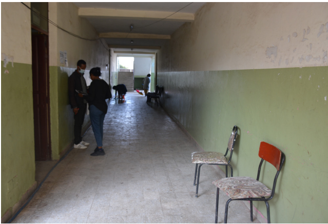
Fig. 75. Insufficient lighting. This hallway has poor lighting, resulting in a dim environment that can cause navigation and way-finding challenges for the users.
