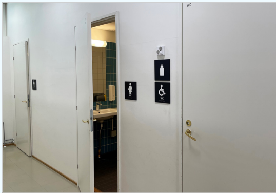
Fig. 25. Clear and contrasting signage is placed on the opening side of the door at the height of 1400–1600 mm.
