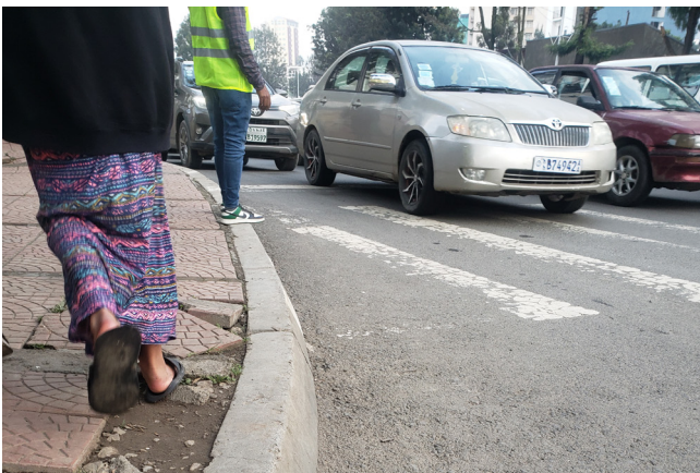
Fig. 34. No curb ramps. The high curb makes transferring between the sidewalk and the street difficult. A curb ramp must be provided to make the crossing safe and accessible.
