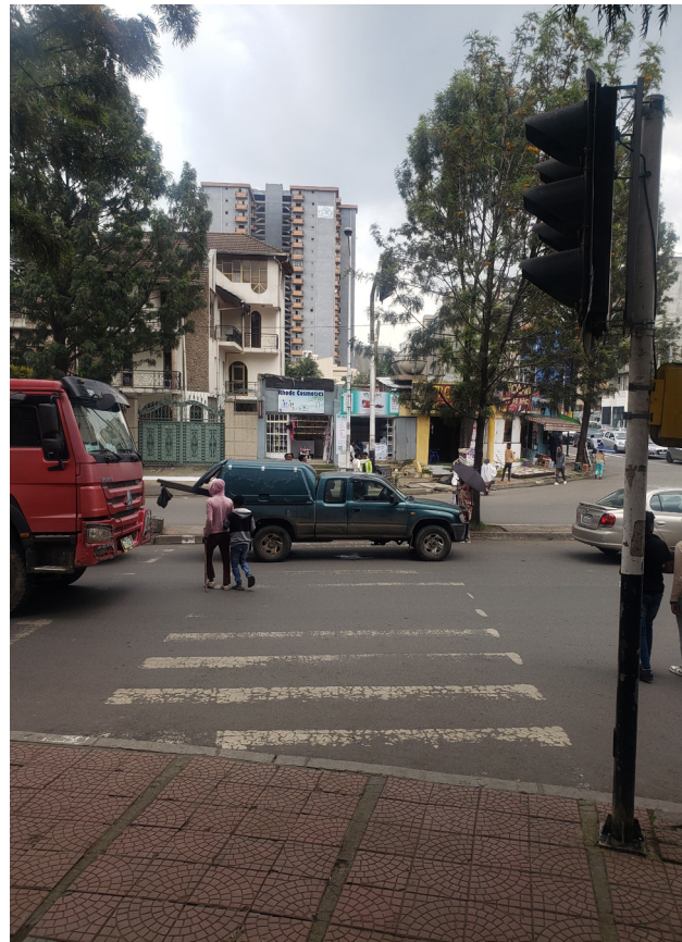
Fig. 35. Unclear road markings. The road markings of this pedestrian crossing are faded and nearly invisible, posing safety risks for pedestrians and drivers alike. There is also a lack of an accessible traffic island and curb ramps.
