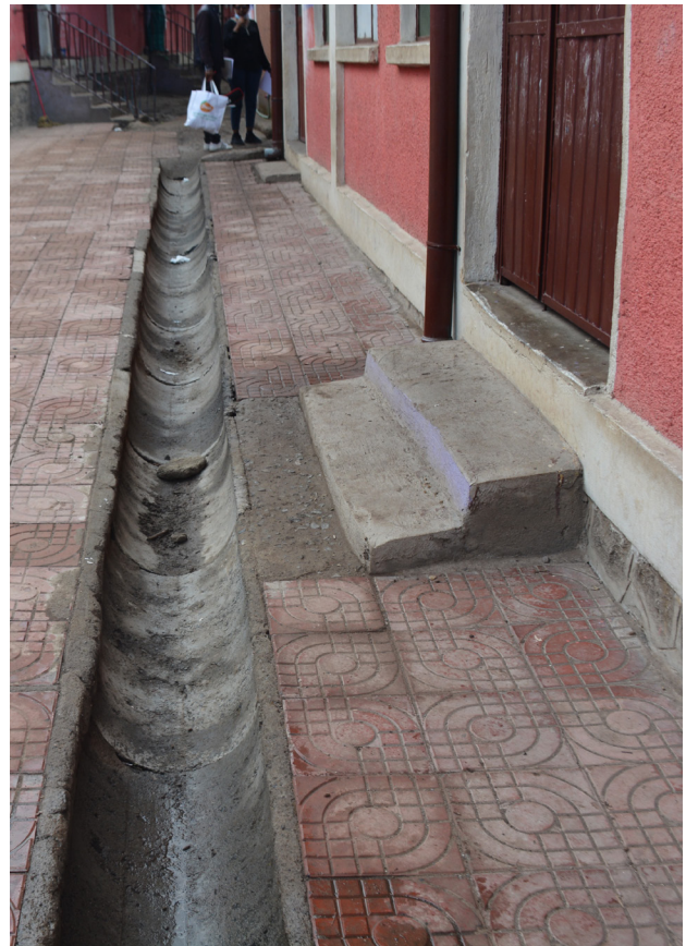
Fig. 58. Inaccessible entrance. This entrance is not suitable for people using mobility aids, and the exposed drainage system along the pathway poses a danger for people with visual impairments.
